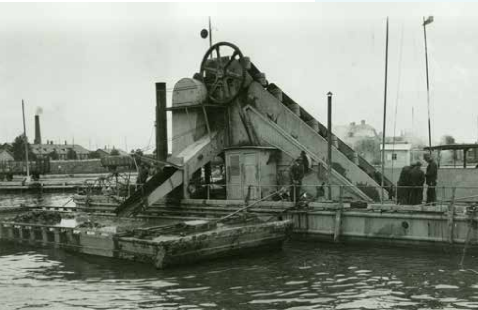
The elevation of the ground and the sludge carried by the River Aura require continuous dredging. Purchased in 1905, bucket-chain dredger Karhu served the Port for more than 80 years. - Turku City archive
