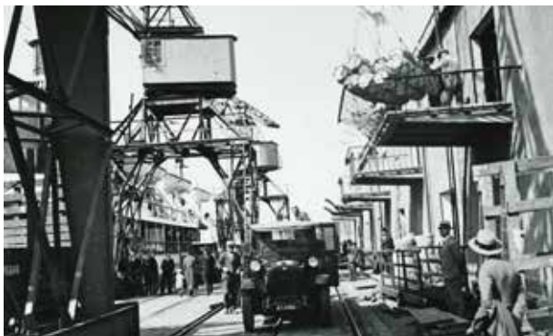
The Butter Magazine built in 1934 was an important factor in stimulating exports through Turku. In addition to providing facilities for testing and storing butter for export, it also helped to generate a flow of other dairy products and foodstuffs. In the picture, the crane is shifting a load of butter in casks called "drittels". – Turku City archive
